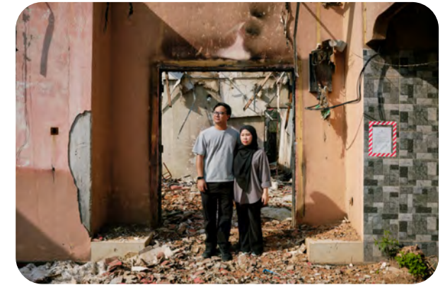
THE AFTERMATH OF THE GAS PIPELINE EXPLOSION IN PUTRA HEIGHTS (MALAYSIA)
